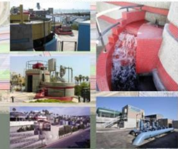
D. STORMWATER RUNOFF RECYCLING FACILITY
