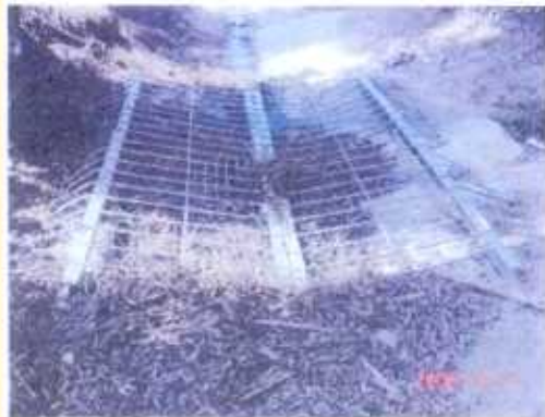
GRATED CATCH BASIN ALONG V-DITCH
