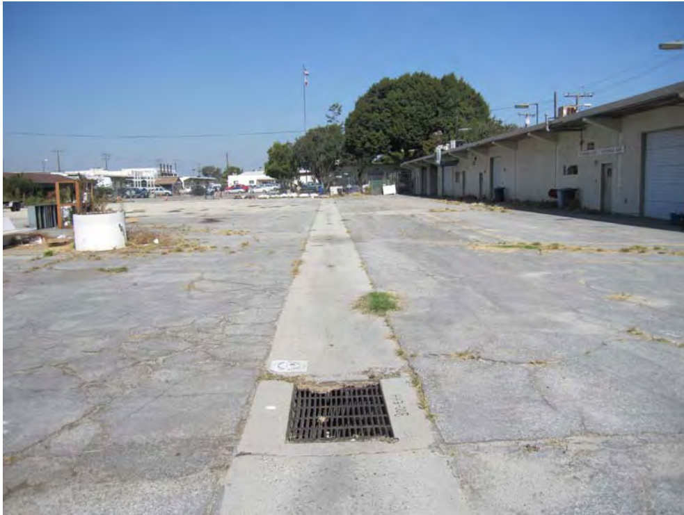
Photo 9. Northerly view of APN 7271-012-904 showing storm drain and abandoned buildings.
