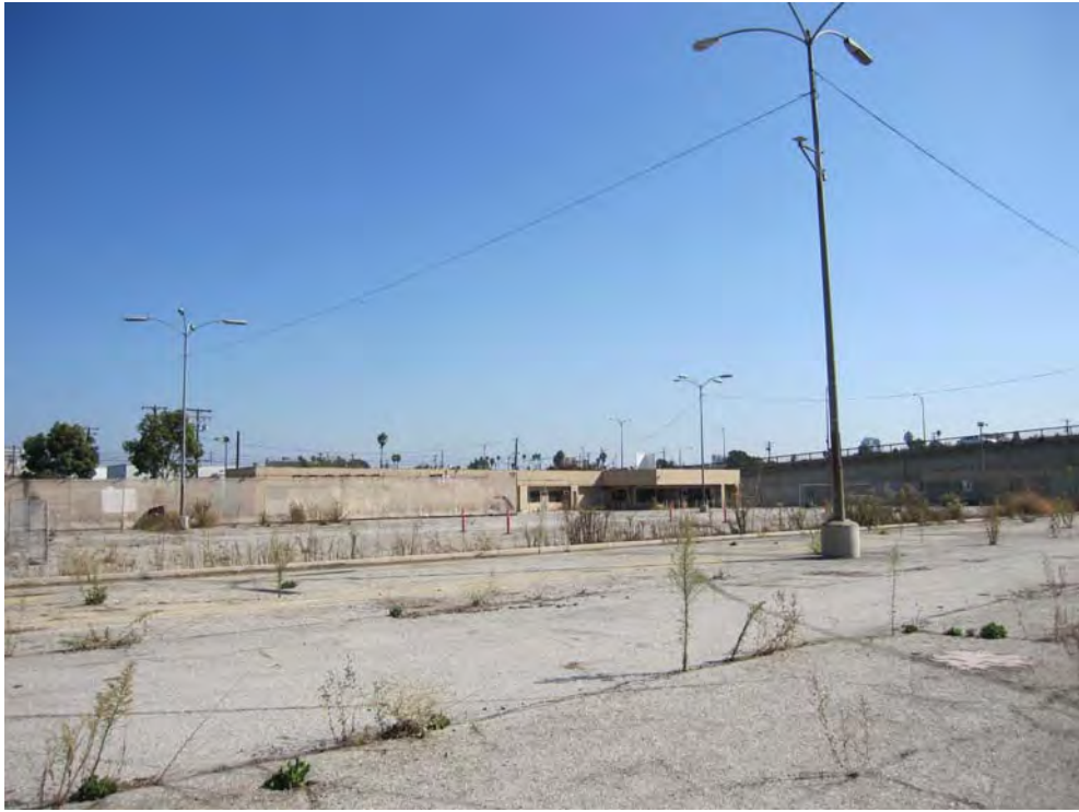
Photo 21. Southeasterly view of the abandoned building on APN 7271-007-903 (901 West Anaheim Street).
