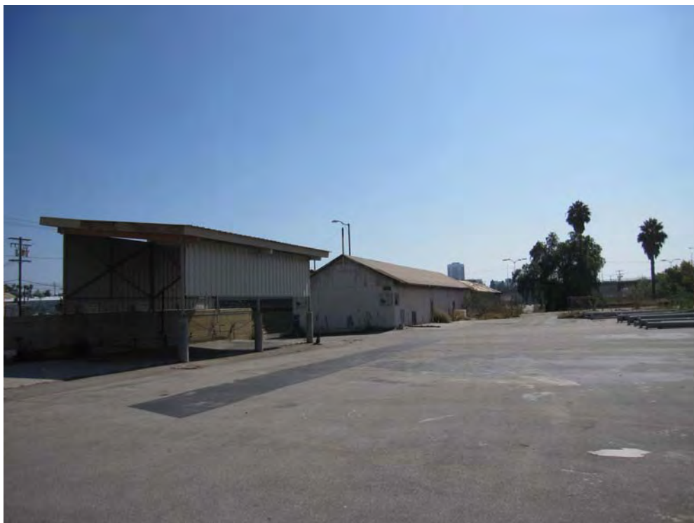
Photo 14. Vehicle Wash Area with Clarifier on APN 7271-008-901.
