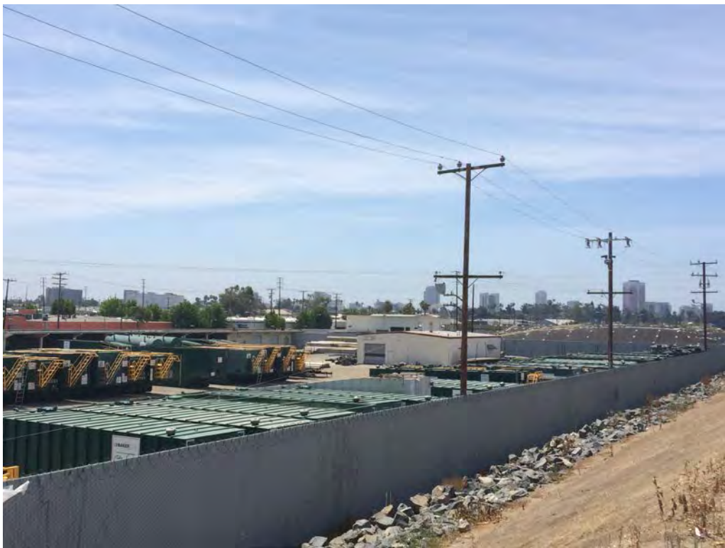
Photo 10. Southeasterly overview of the Baker Yard portion of the Property.
