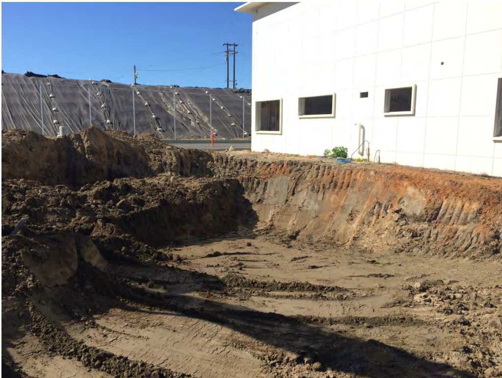
Photo 2. Excavation of area beneath former historical building.
