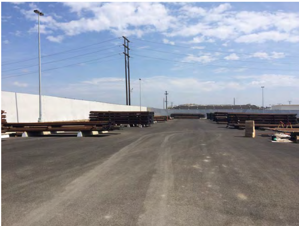
Photo 6. New portion of the Petros Yard recently remediated by removing refuse and lead-contaminated soil.
