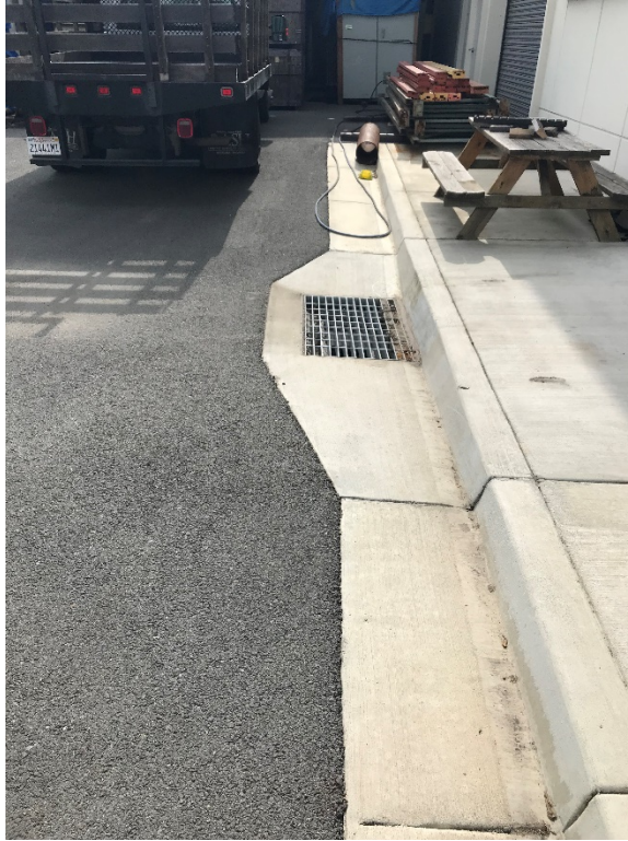
Photograph 1: Surface Drains at Property
