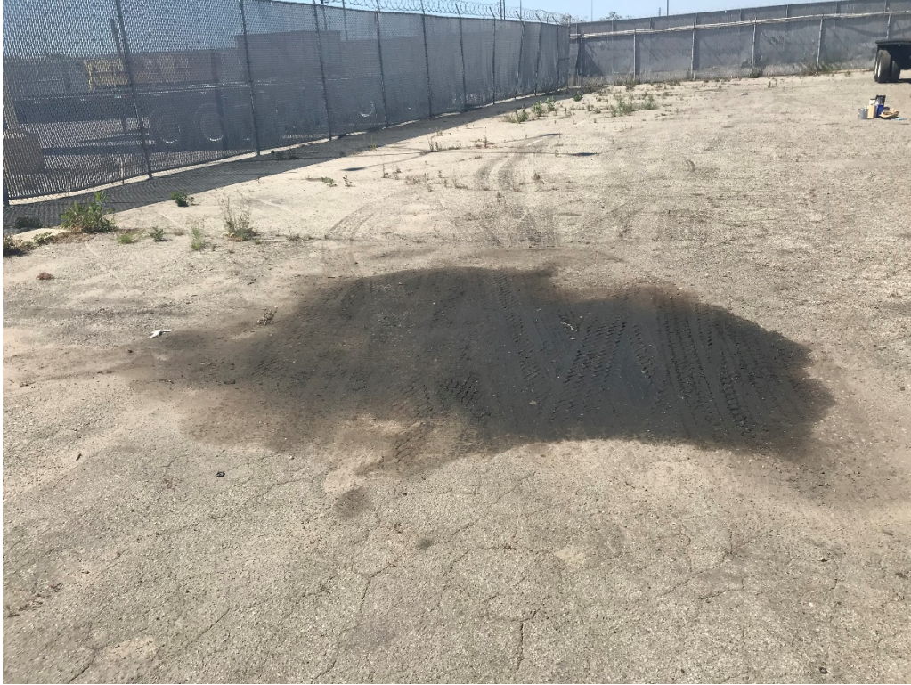
Photograph 19: Staining at 929 West Anaheim Street
