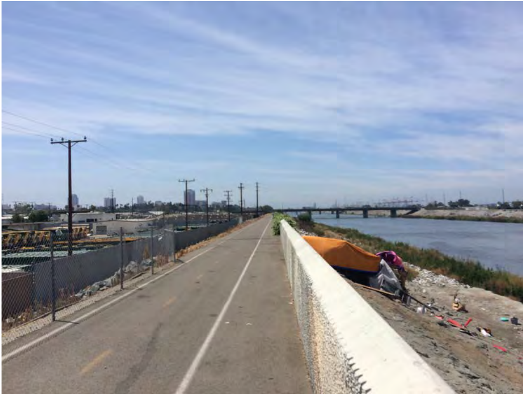
Photo 15. Southerly view of the river trail and LA River adjacent to the west of the Property.
