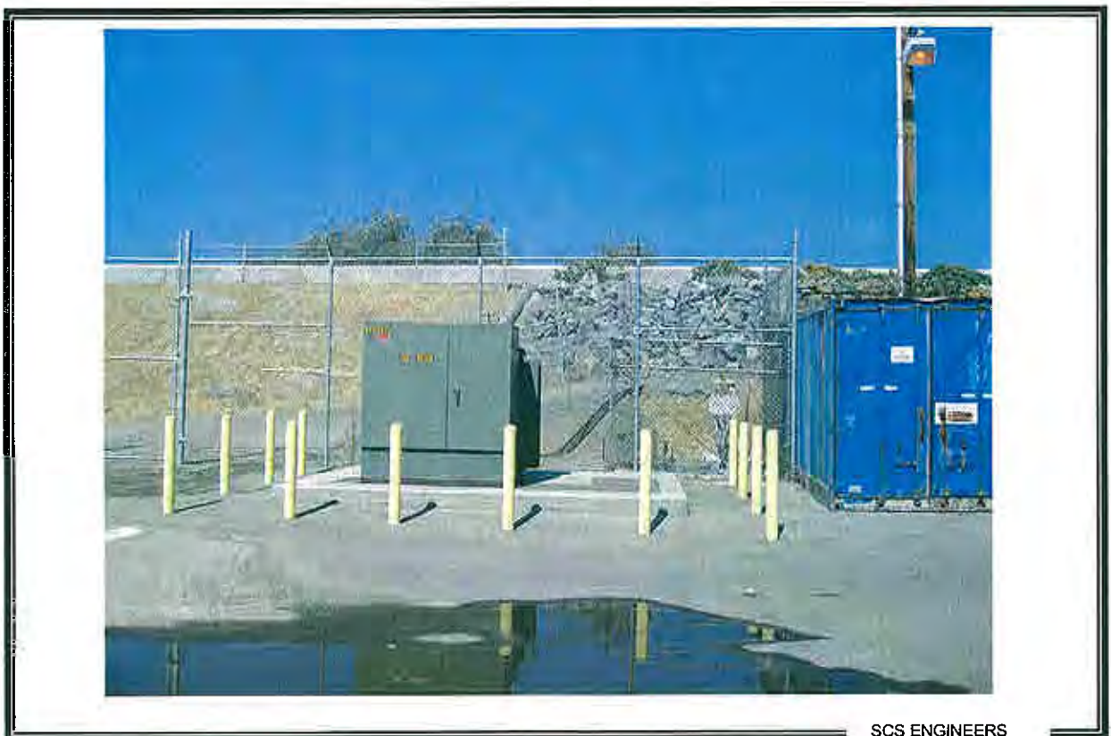
Photo 14. SCE Pad-mounted Transformer North of the Pump Station
