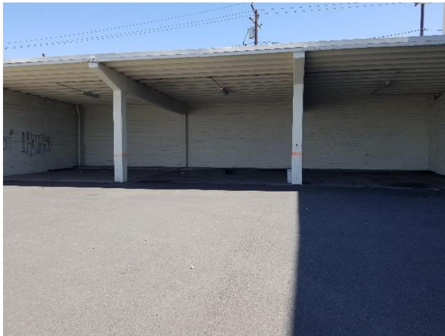
Covered Parking that Adjoins Main Building to North (View East)
