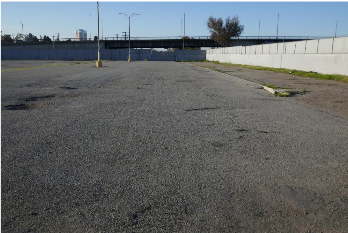
Photograph 6: 929 Anaheim Street property, looking south, March 29, 2021.
