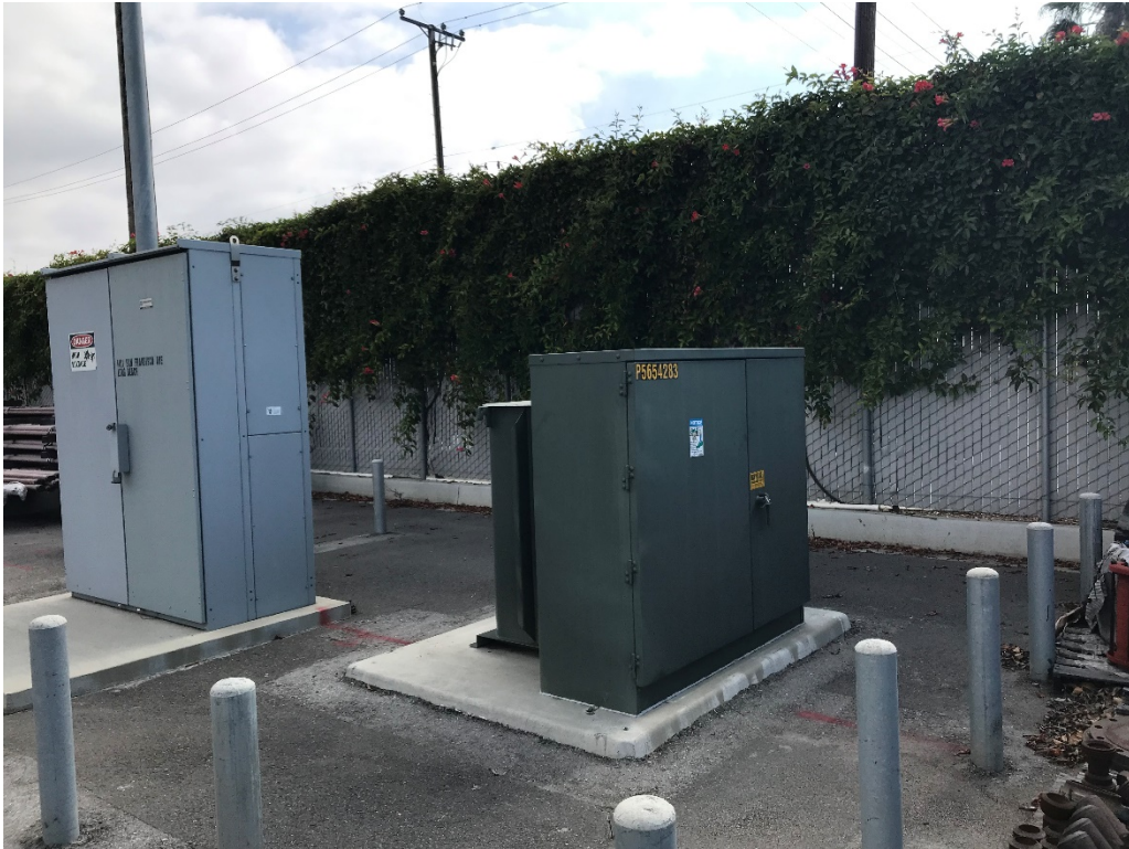
Photograph 7: Pad-Mounted Transformer
