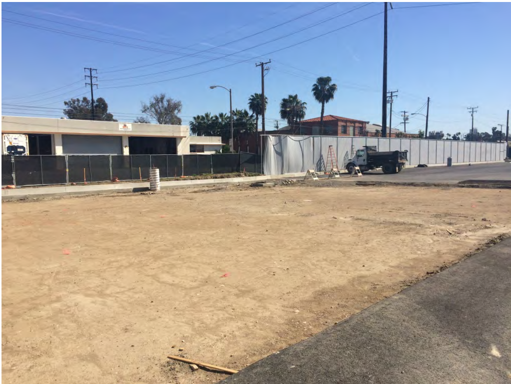
Photo 4. Completion of backfill of historical building area on Yard Parcel.
