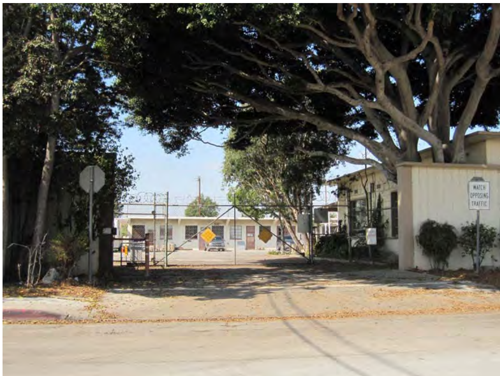
Photo 4. Westerly view of the Property at 1601 San Francisco Avenue where the 16 th Street right-of-way traverses the Property (this area was not accessible for inspection).
