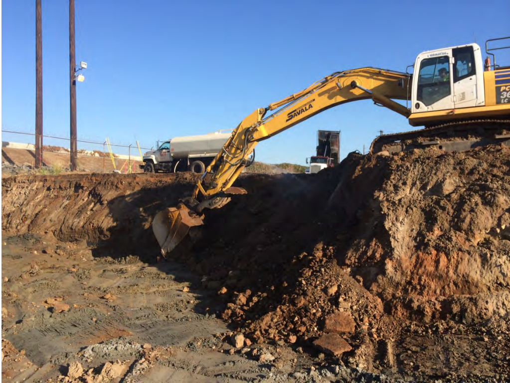
Photo 1. Excavation of lead-impacted soil with debris down to native soil.
