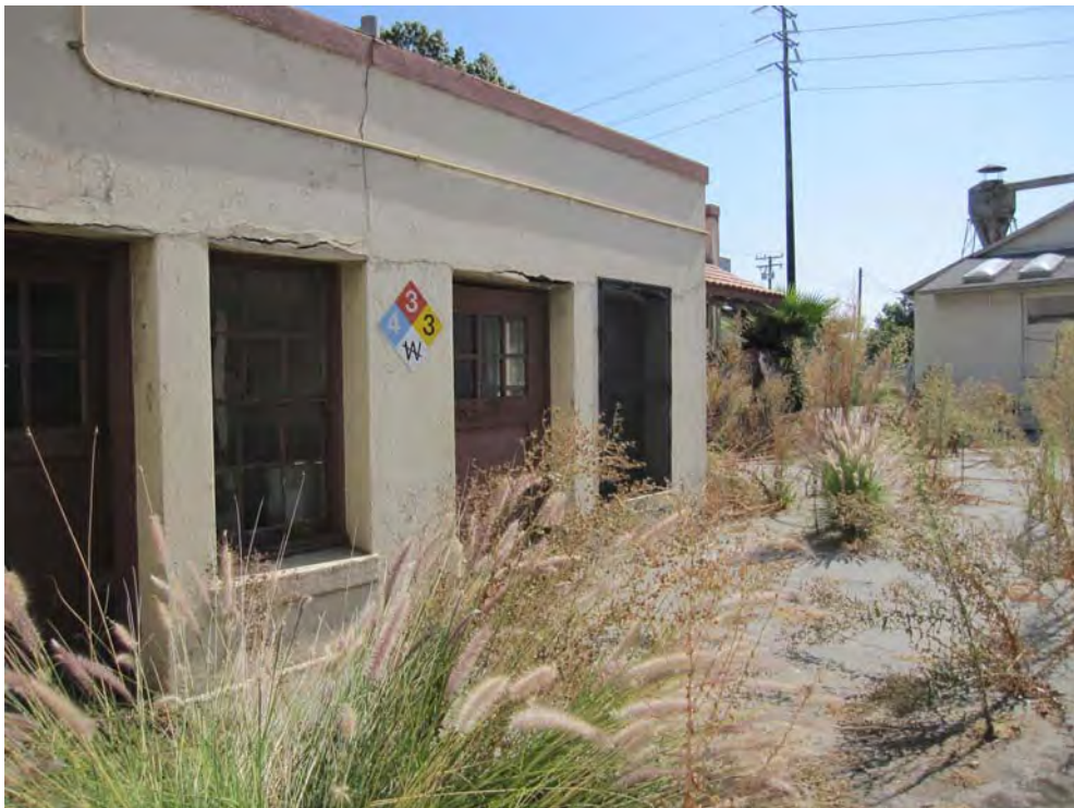
Photo 12. Vies of abandoned chemistry lab building on APN 7271-011-900.
