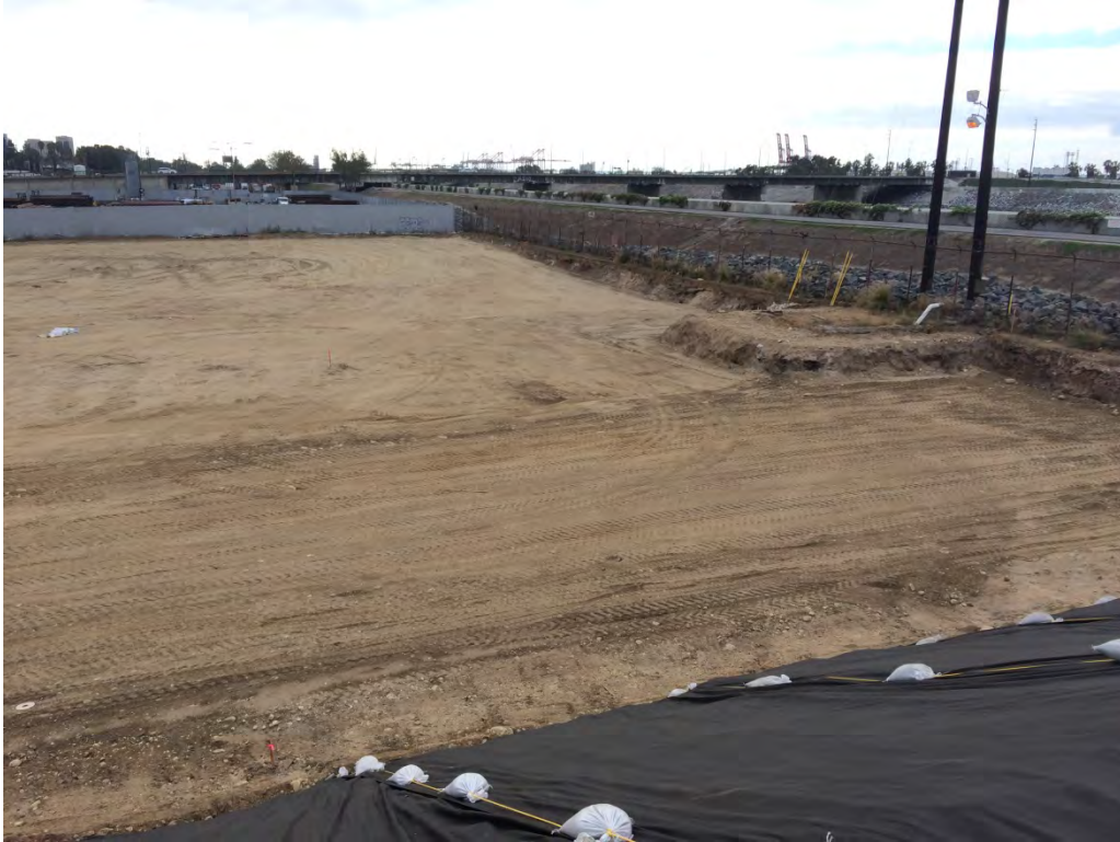
Photo 3. Completion of backfill of excavation on southern portion of Yard Parcel.
