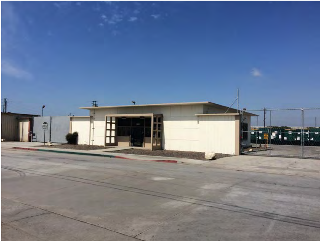
Photo 9. Structure at Baker Yard portion of the Property.
