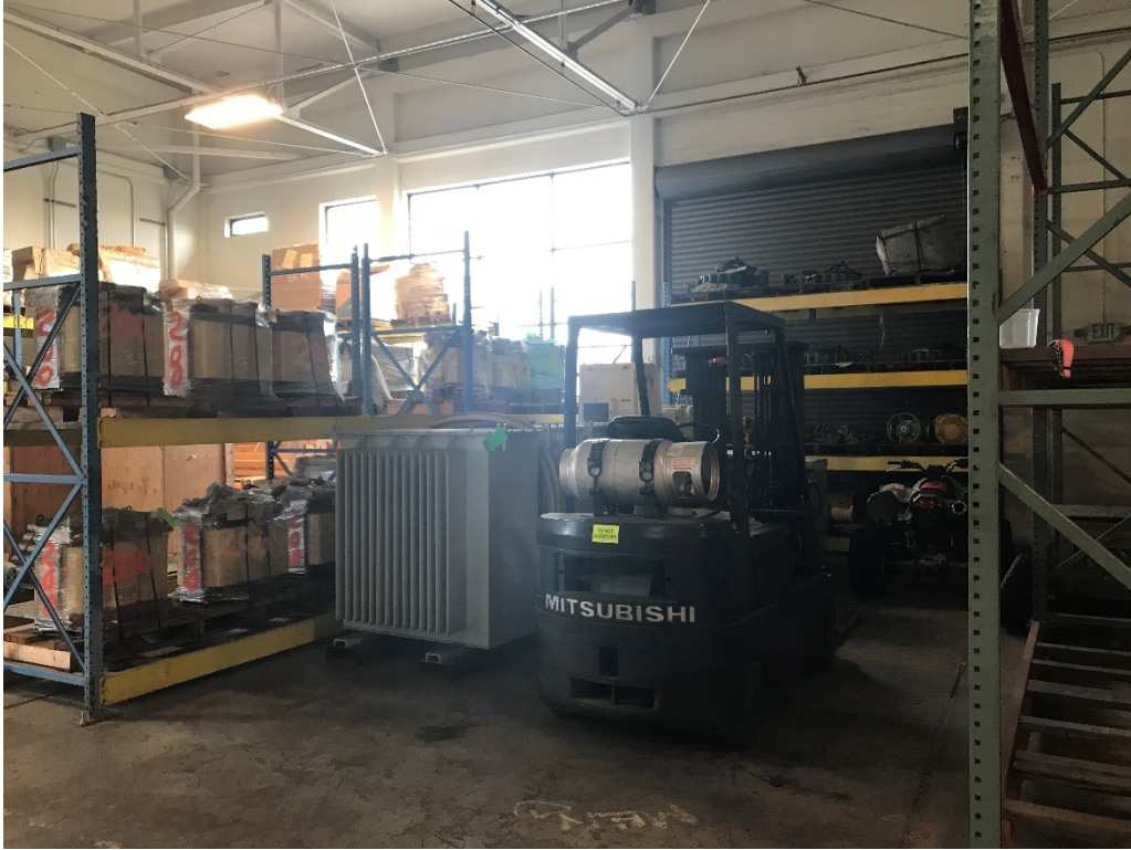
Photograph 9: Forklift Located inside Concrete Building
