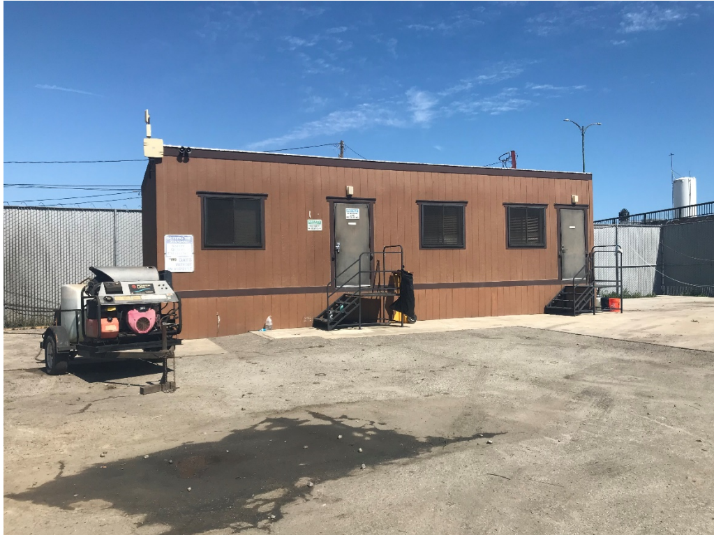
Photograph 16: Trailer and Staining at 929 West Anaheim Street
