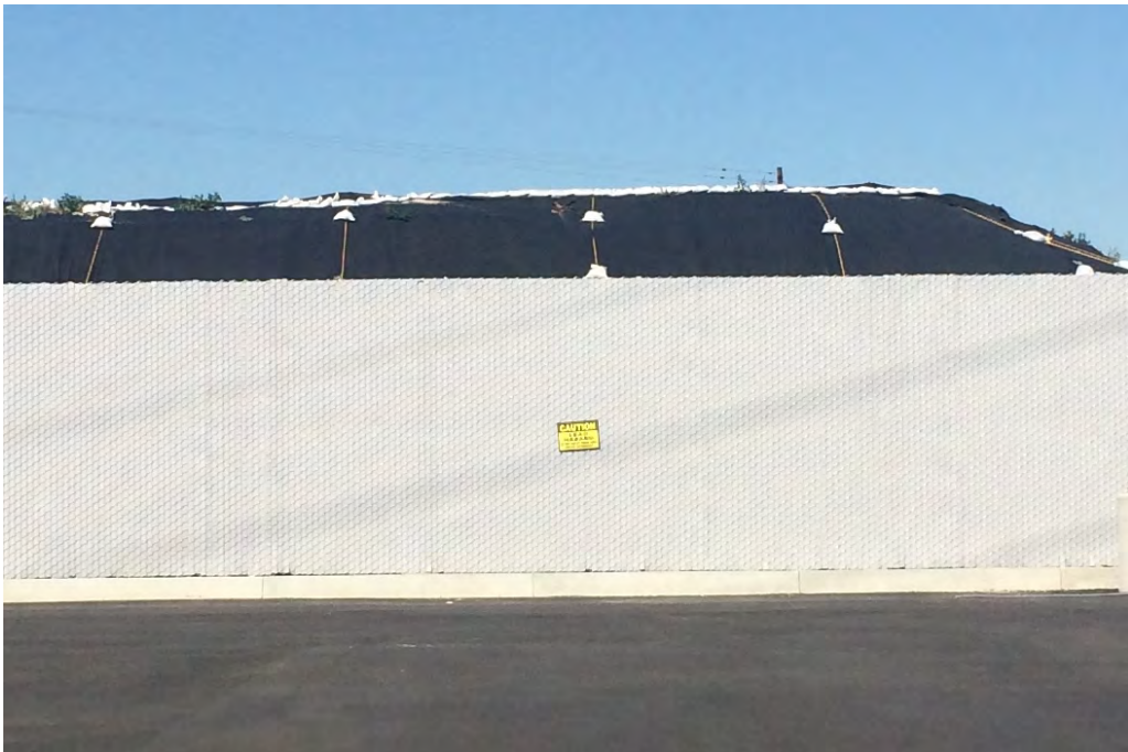
Photo 6. View of privacy fencing bounding south side of AOC (Long Beach Parcel) with Lead Hazard sign.
