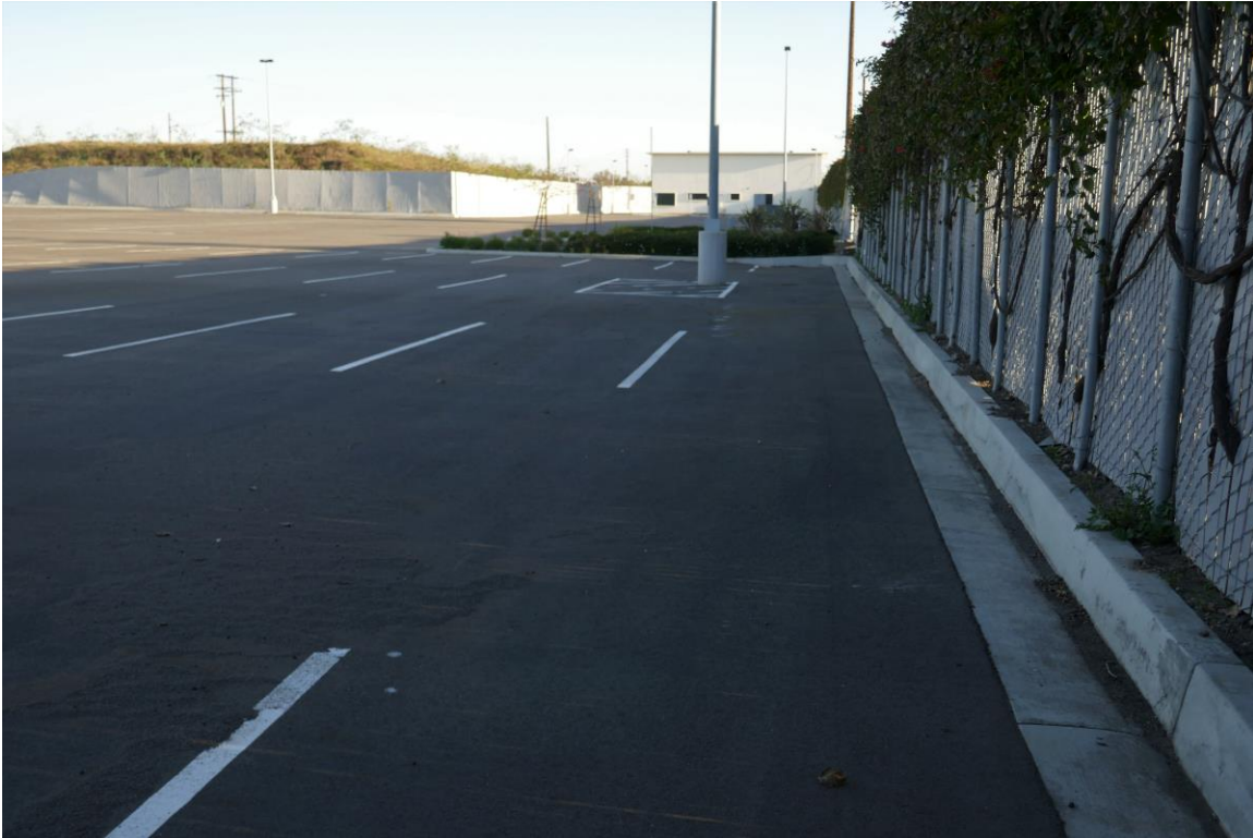
Photograph 3: 1401 San Francisco Avenue property, looking north, March 29, 2021.
