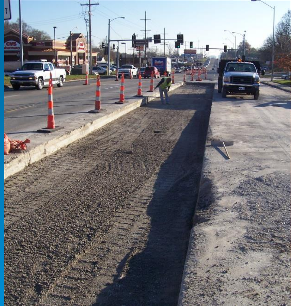
Typical Open Cut Construction Work Area Photos courtesy of Black & Veatch, 66" steel water pipe
