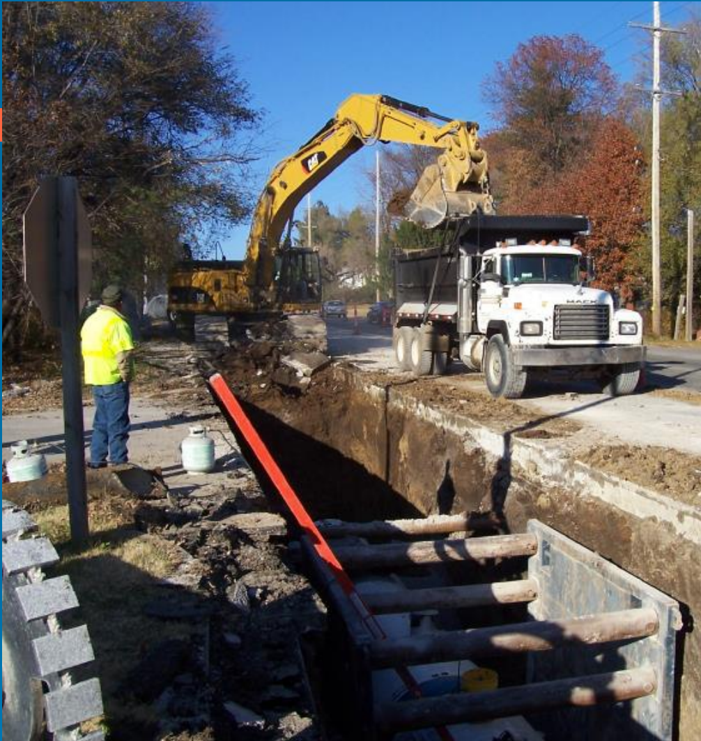
Typical Open Cut Construction Work Area Photos courtesy of Black & Veatch, 66" steel water pipe
