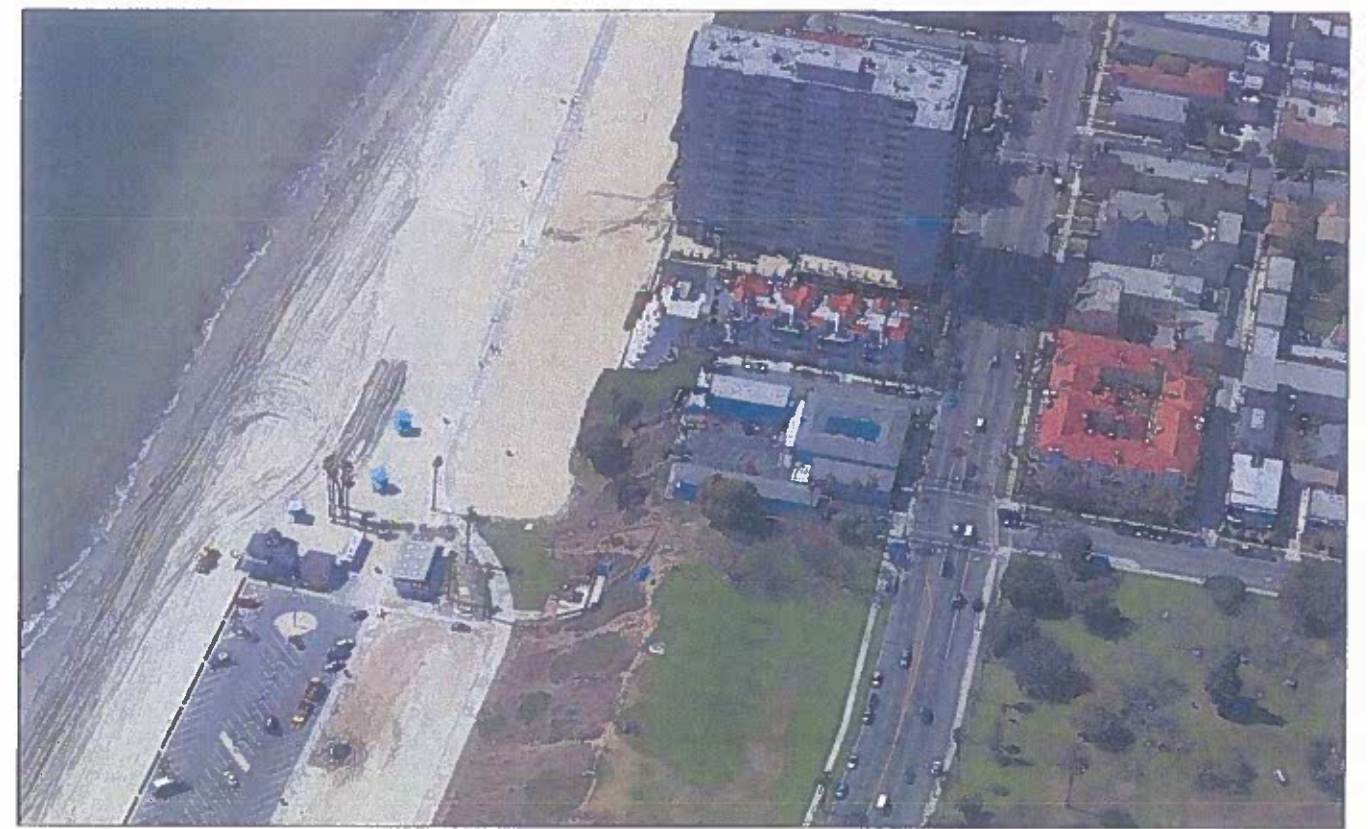
Aerial view looking West
