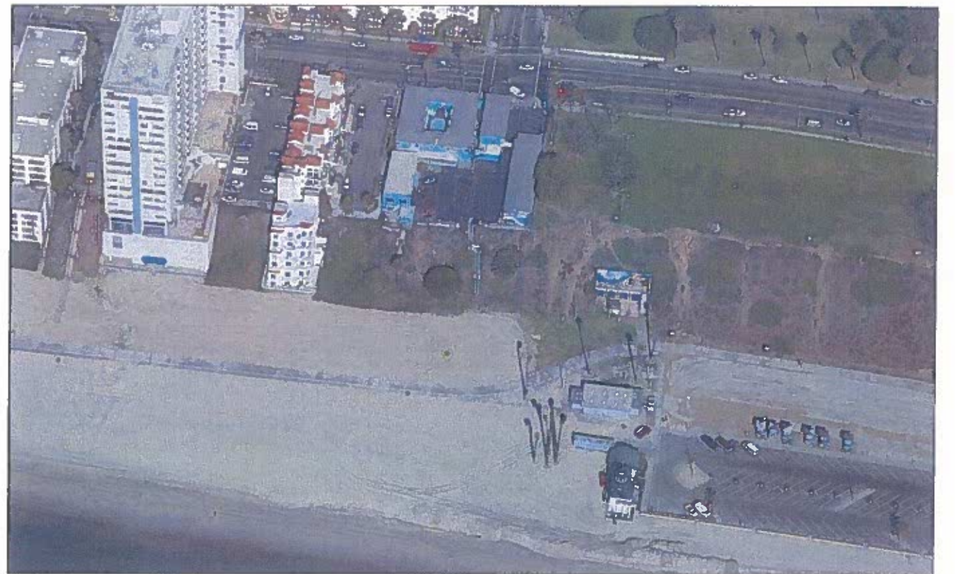
Aerial view looking North
