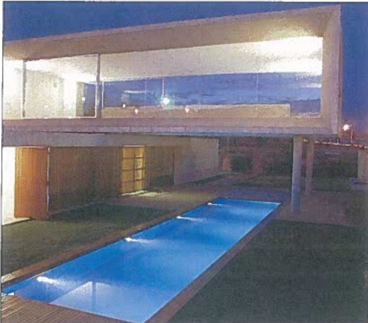
Building supported by piers
