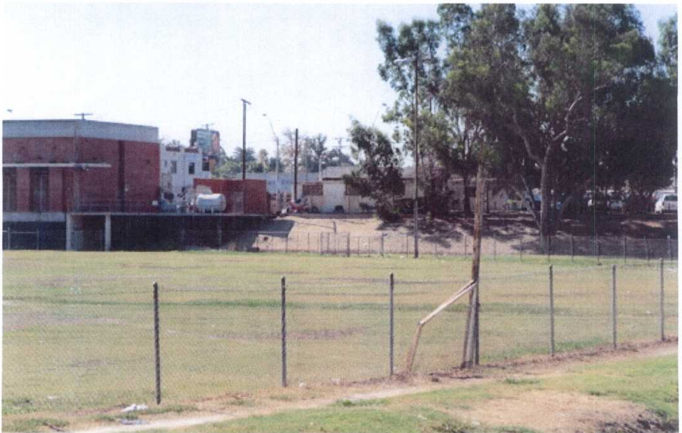
• Pump Station – looking South at PCH
