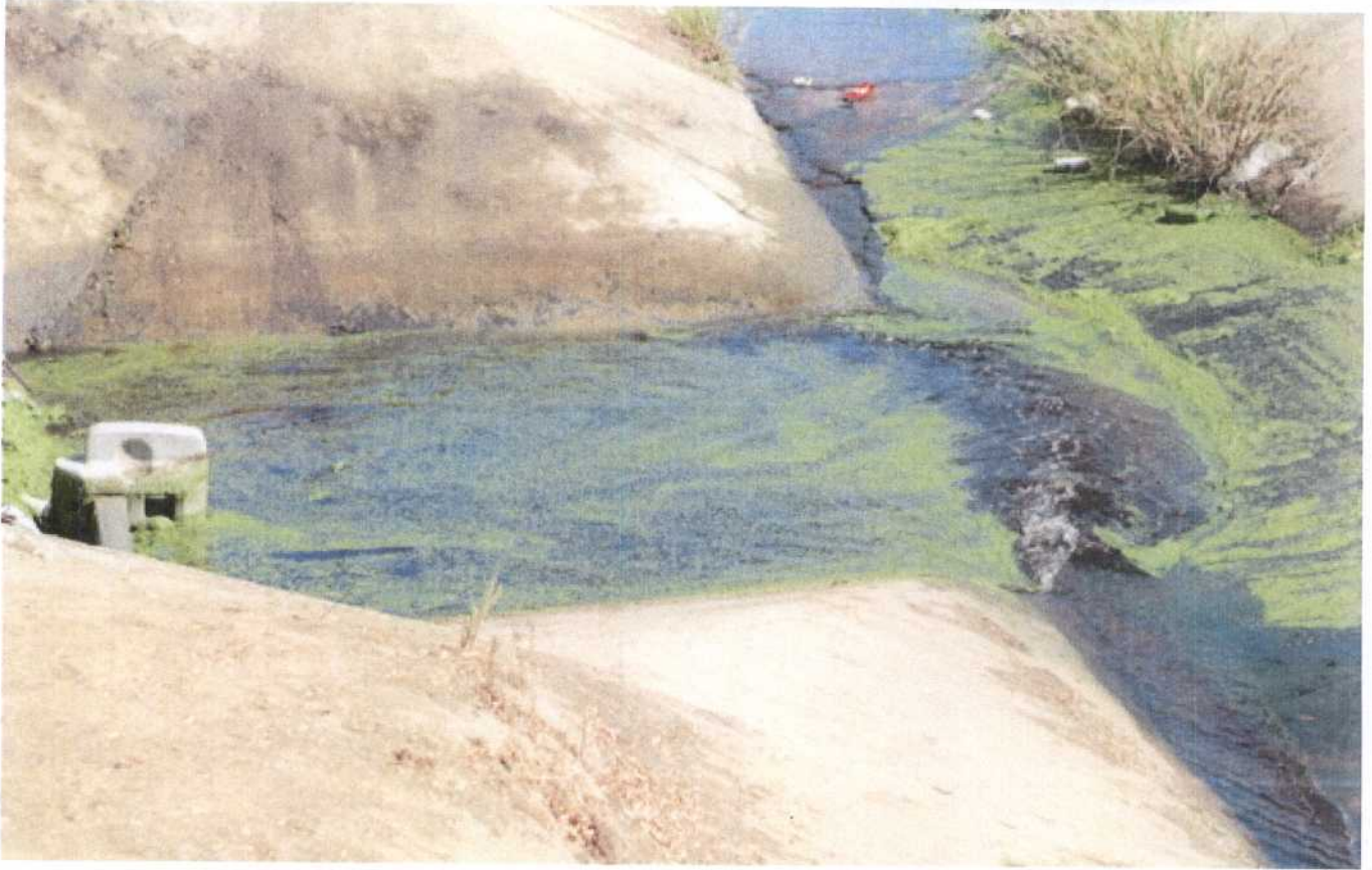
• Current Drainage System condition
