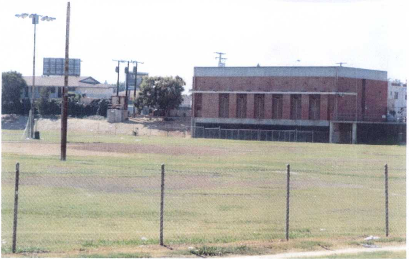
• Pump Station – looking South at PCH
