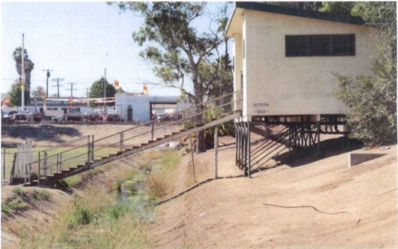
• Pump Station on Walnut Ave. – looking South at PCH
