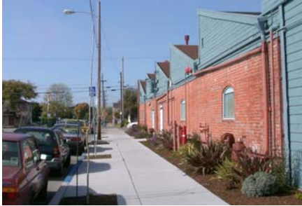
Westside’s economic strategy could include industrial studios for commercial artists as it exists in West Berkeley Industrial Area
