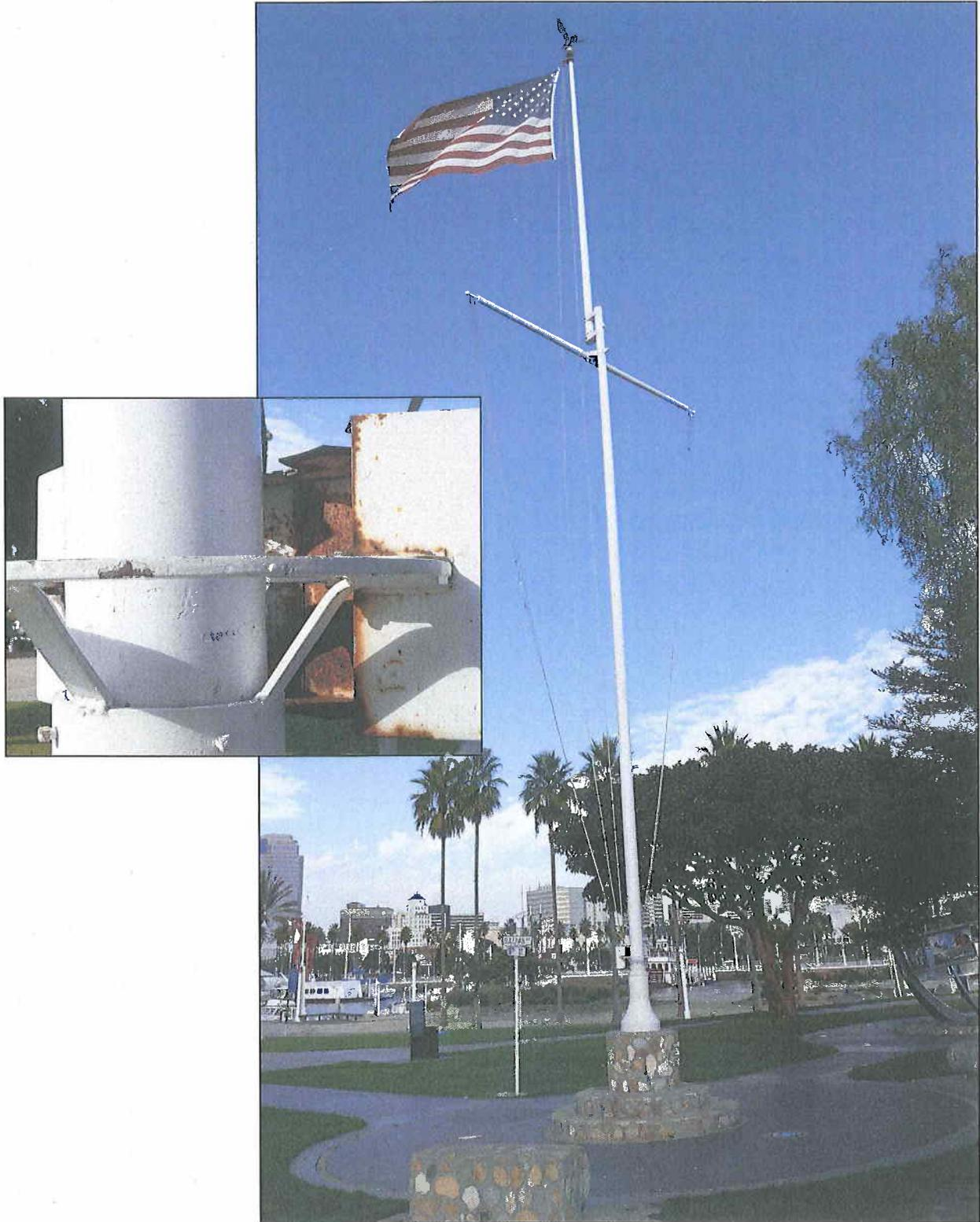
Ship mast will be rigged with new rope and the rusted areas sanded, primed and the mast repainted.
