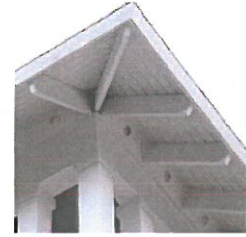
9 Eifs Exposed Rafter Tails
