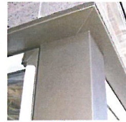
18 Brake Metal Wrapping over Steel Tube
