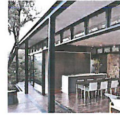
12 Exposed Steel Columns / Beams
