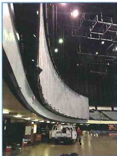
The tension grid is augmented by a system of movable drapes hung from a surrounding truss that screen off the permanent, arena-style seating sections.
