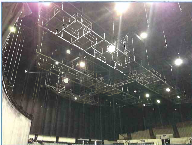
The nine-section elliptical tension grid can be lowered from the high steel to any desired operating height.
