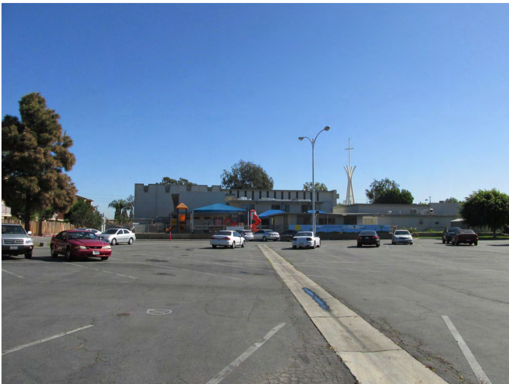
Photograph 2. Church looking west from rear of parking lot.
