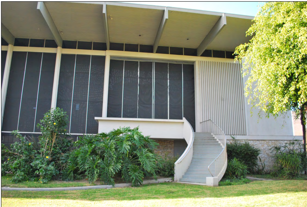
Photograph 2. Chapel – outdoor balcony connected to interior preaching pulpit
