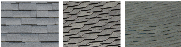
Composition shingles in an appropriate color, like the above examples, would be acceptable for a Minimal Traditional residence. Shingles should be in a darker, neutral color, but not so dark as black.
