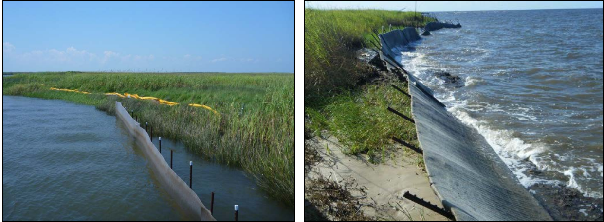
Figure 3-3. Shoreline barriers used during the Deepwater Horizon oil spill. Filter fences require many stakes. Usually there is not enough time to deploy this type of barrier after a spill, they have limited effectiveness, and they are difficult to remove. The hard boom has become stranded on the marsh. Photo credit: Helen Chapman (left); Thomas Minter (right).
