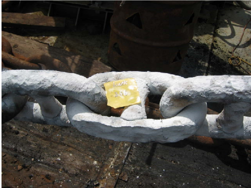
Figure 7-2 Bacterial corrosion (DNV classed FPSO offshore West Africa).
