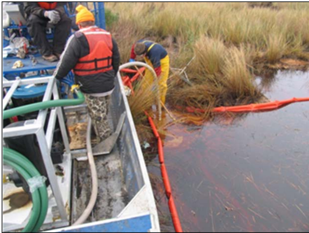
Figure 3-7. Vacuuming of thick oil from the water surface in a marsh channel, Bayou Perot, Louisiana in February 1997. Photo credit: Jacqueline Michel.
