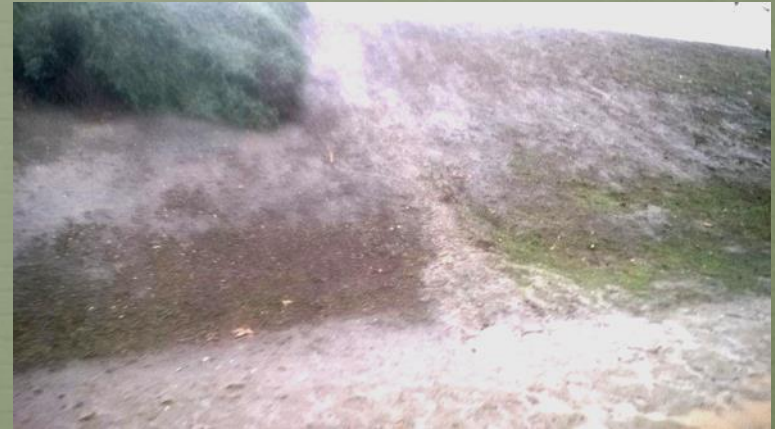
LA River Levee Run-off
