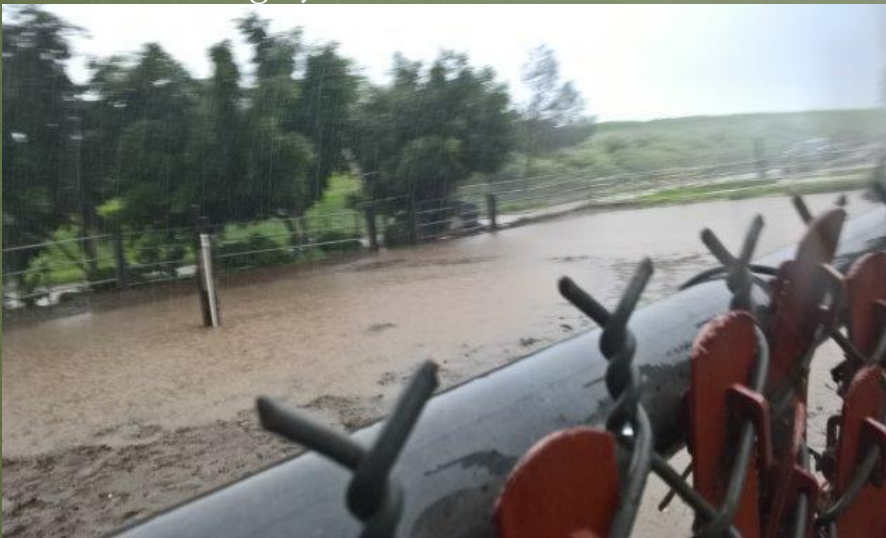
Run-off Toe of the Levee and From the Horse Trail Flowing From the North
