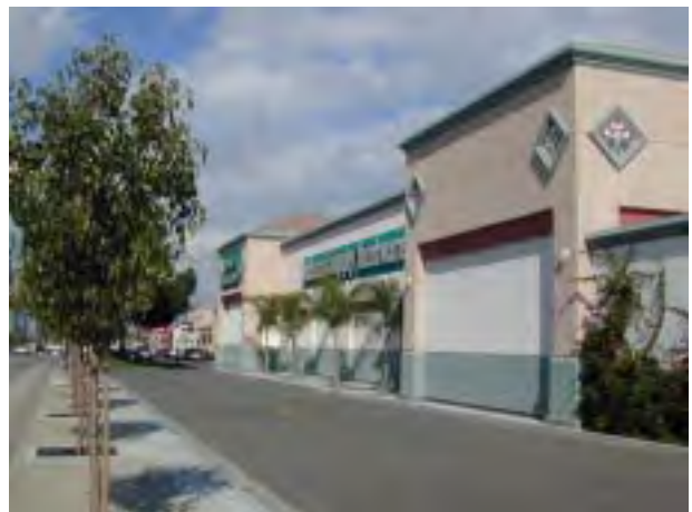
OSH Store in shopping center: blank wall facing Atlantic Avenue
