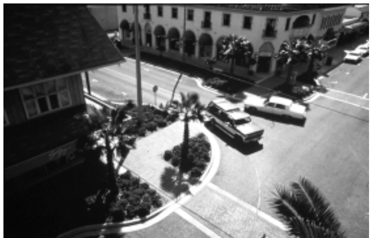
Example of a bulb-out at a street intersection
