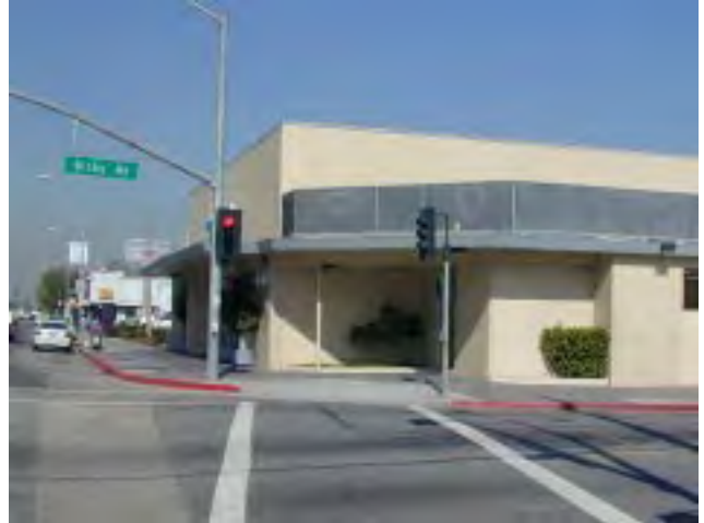
The Bank of America building with the corner blocked off. The entrance should be located at the corner with glass windows that allow views into the bank.
