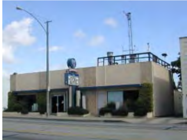
Exposed roof equipment is prohibited.
