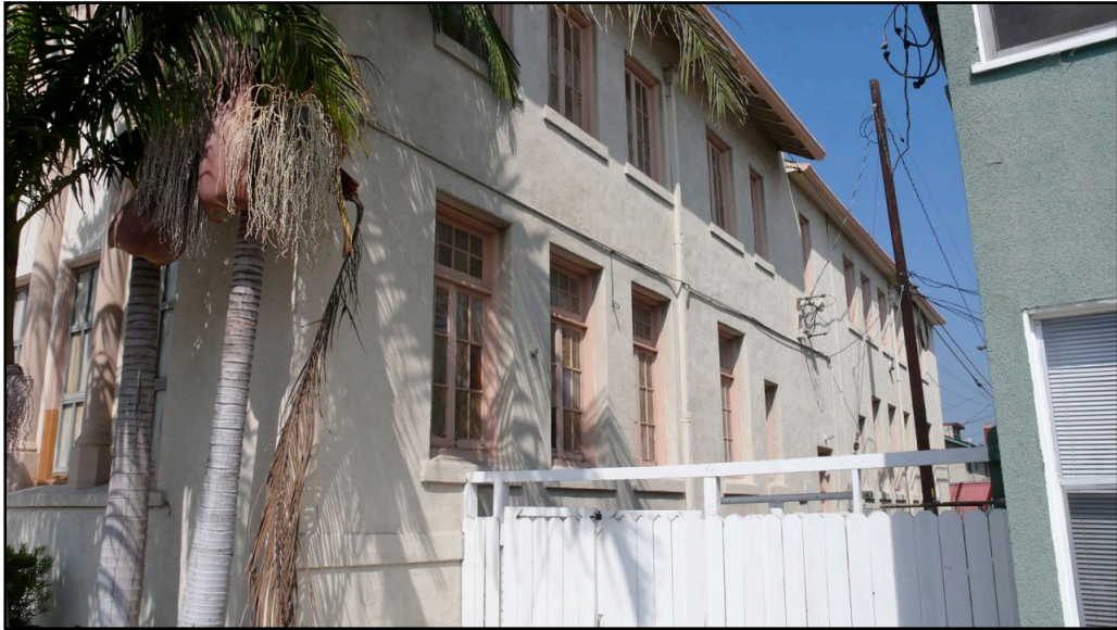
Photo 5. 3215 E. 3rd Street, eastern elevation. [9-26-2012]
