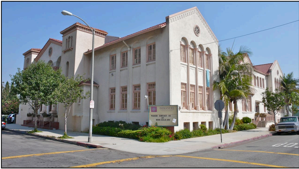
Photo 1. 3215 E. 3rd Street, western and southern elevations. [9-26-2012]
