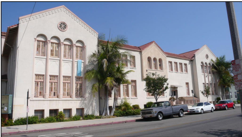
Photo 3. 3215 E. 3rd Street, southern elevation. [9-26-2012]
