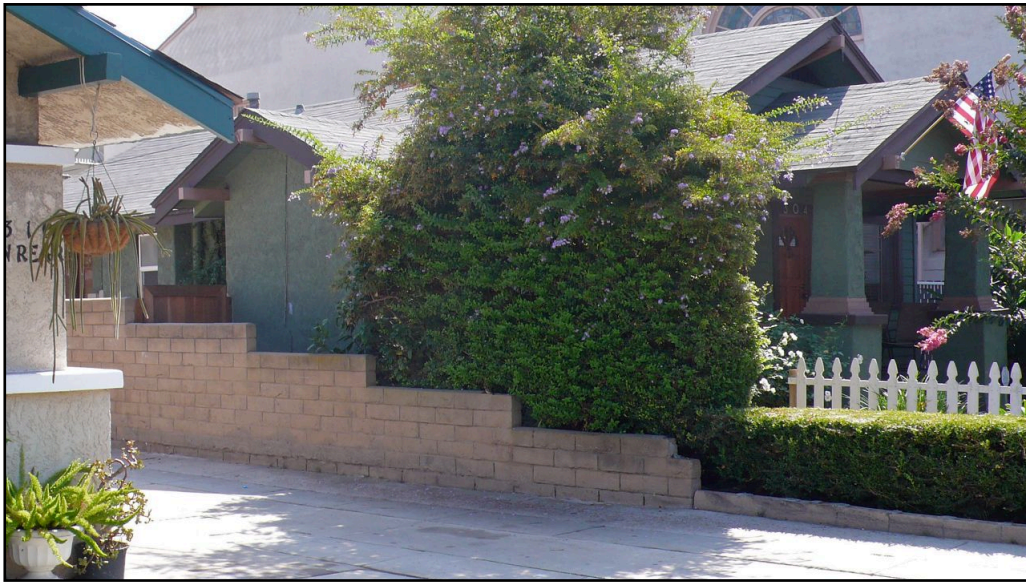
Photo 7. 302 Obispo Avenue, northern elevation. [9-26-2012]
