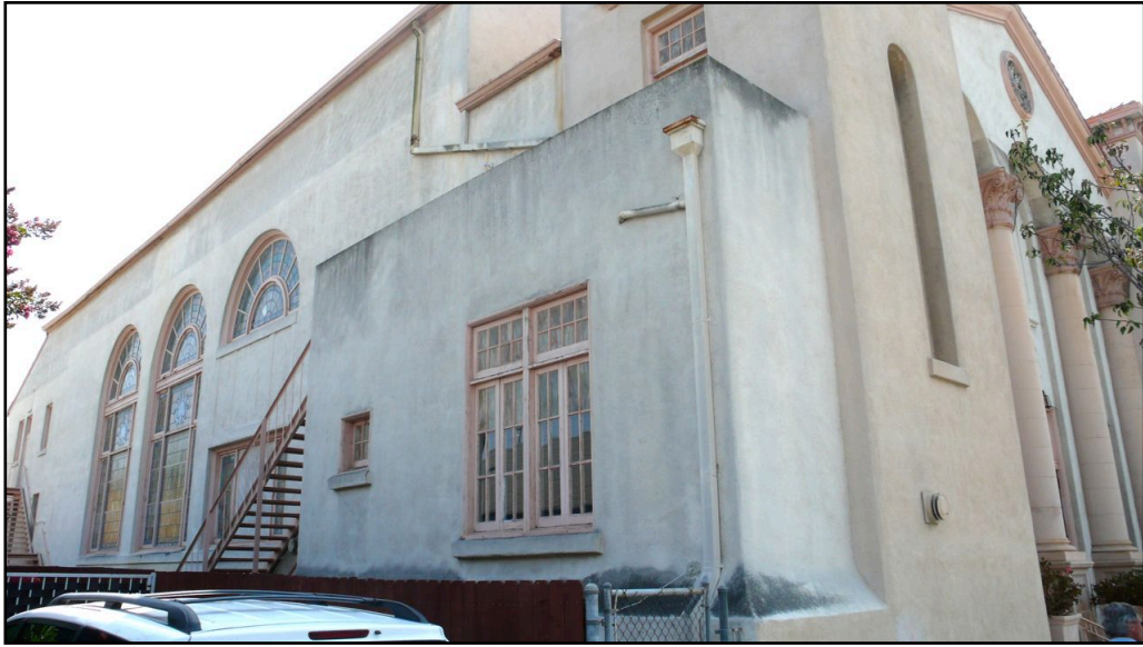
Photo 4. 3215 E. 3rd Street, northern elevation. [9-26-2012]
