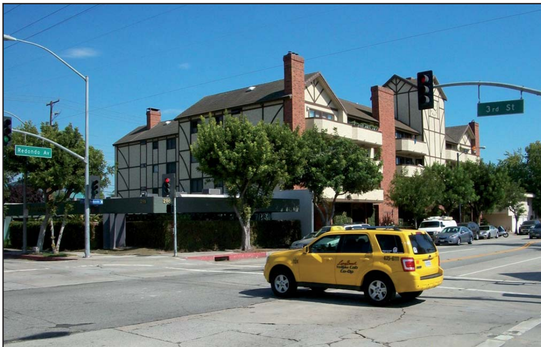
Photo 4 - Commercial building at southeast corner of East 3rd Street and Redondo Avenue.
