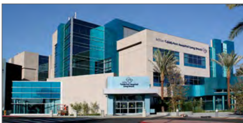
The corridor contains a wide variety of single- and multifamily housing, commercial and service businesses, and medical facilities.
