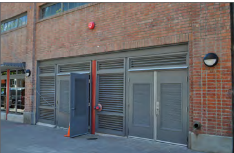
Utilities should be outside of the public right-of-way and should be screened.
