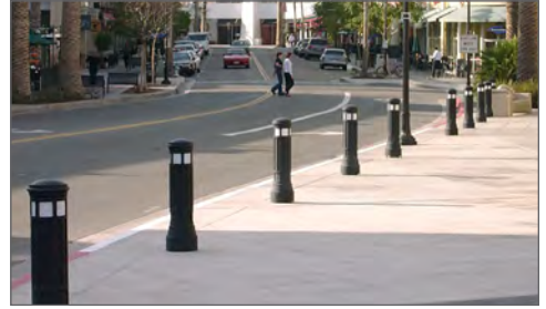
Lighted bollards provide pedestrian-scale lighting by illuminating a safe path of travel.
