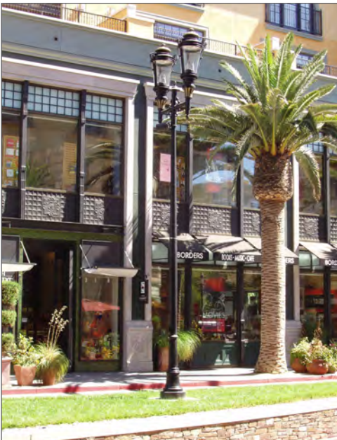
Light poles should be out of the public right-of-way and should be a similar style with the architecture of surrounding buildings.
