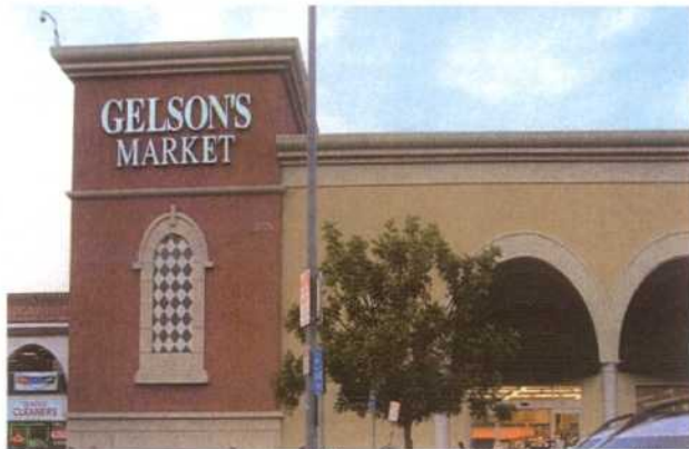
Signage well placed on building.
