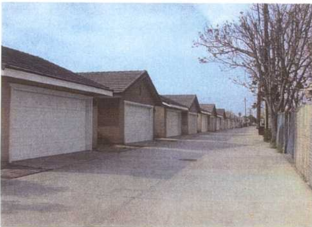
Front doors visible from the street (top); parking hidden behind (bottom).
