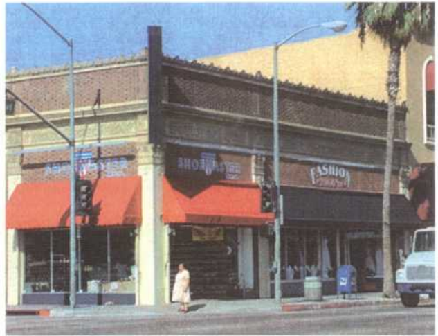
After façade rehabilitation.
