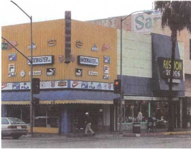
Before façade rehabilitation.
