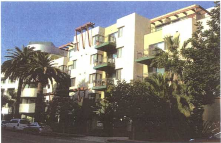
Recently built mid-rise mixed-use and housing development in a contemporary style.
