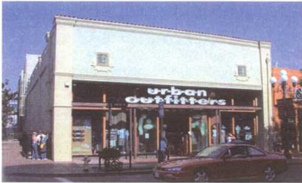
A single tenant in a small building might create a single continuous bay.
