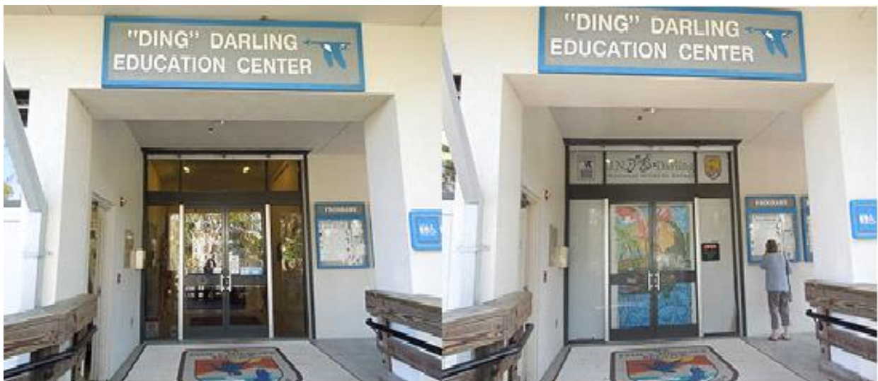
A bird friendly film was applied at the entrance of the Ding Darling Education Center at the J. N. "Ding" Darling National Wildlife Refuge. Photo shows entrance before (left) and after (right) application. Photos by USFWS
