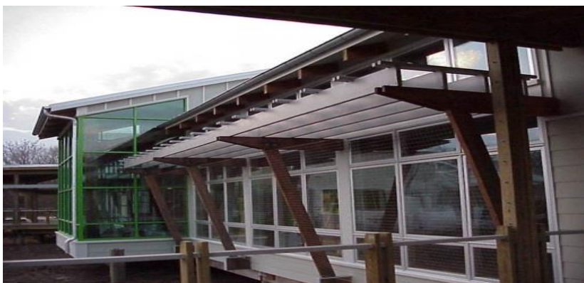
Window netting installed feet from window on slanted wooden beams. Photo by USFWS
