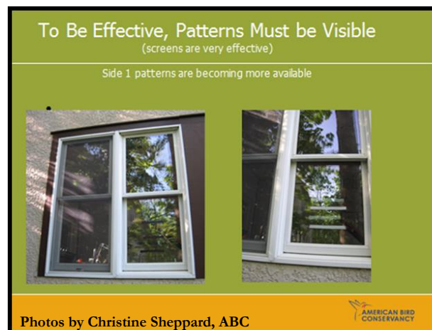
The image shows how pattern spacing on glass can work to deter birds. Images by ABC and Roy Hancliff
