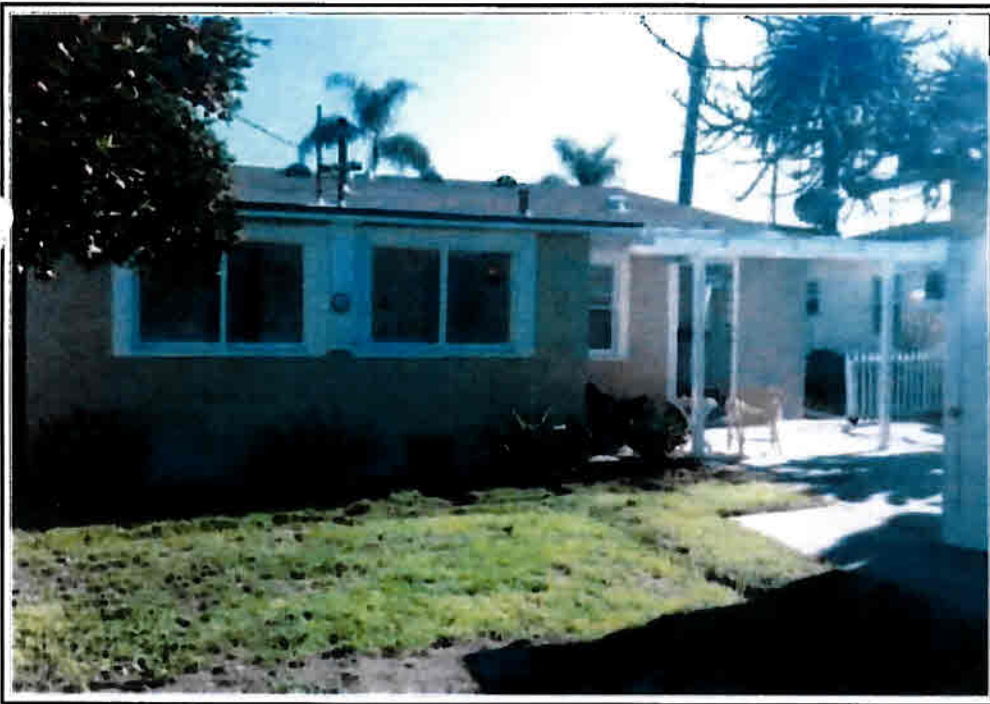
REAR OF SUBJECT PROPERTY
