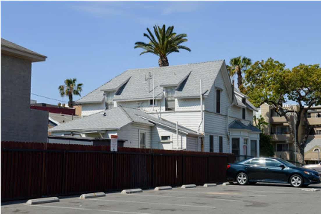
Parsonage Residence, East Elevation, View Southwest, Photo: 2017.
