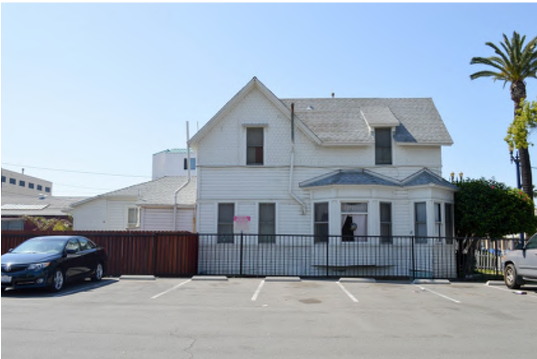
Parsonage Residence, North Elevation, View South, Photo: 2017.
