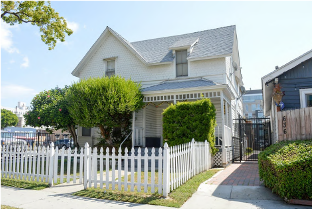
Parsonage Residence, Primary Elevation, View Northeast, Photo: 2017.
