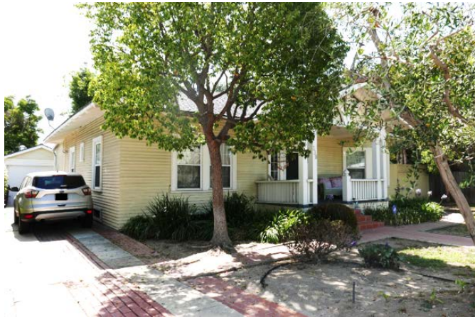
Northern and Primary (Western) Façade, 338 Junipero Avenue
