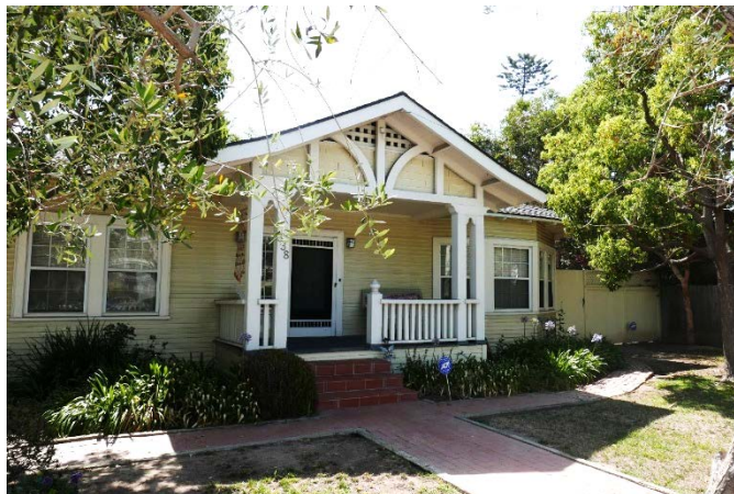
View of Primary (Western) Façade, 338 Junipero Avenue
