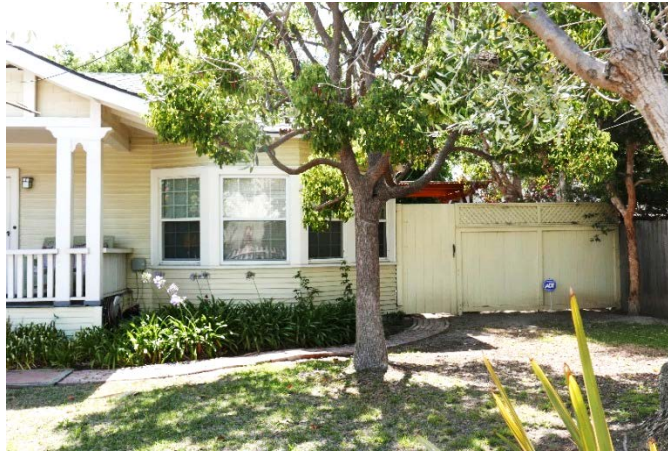
Detail of Primary (Western) Façade, 338 Junipero Avenue
