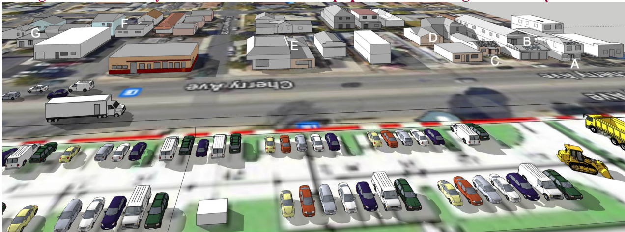
Figure 5 – Proximity between Construction Equipment or Parking and Nearby Homes
