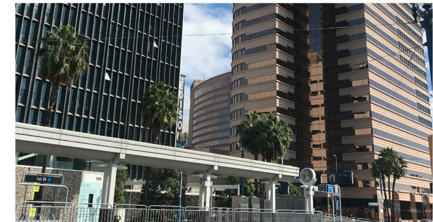
9 VIEW LOOKING SOUTHEAST ON FACING COMERICA BANK BUILDING
