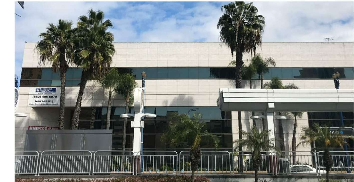
8 VIEW LOOKING EAST ON LONG BEACH BLVD. FACING BOA BUILDING
