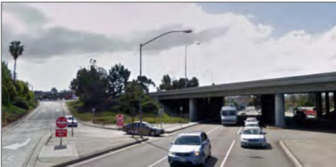
Traveling southbound from the off-ramp at Long Beach Boulevard requires a cautious left turn across northbound traffic, which includes cars, buses, and trucks.
