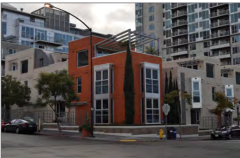
High quality materials are encouraged for residential buildings. Windows should allow for a shadow line and depth.
