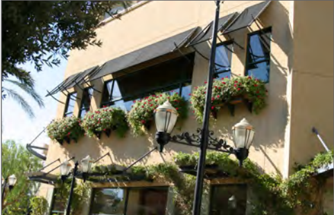
Solar orientation of the building, overhangs, and other devices placed on the exterior of buildings reduce direct sunlight into interiors, lowering heat gain and the amount of energy needed for cooling.
