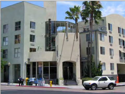
Special attention should be paid to corner features of buildings at prominent intersections.
