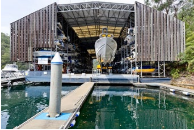
Well-designed boat storage facilities should screen views of service areas. Photo Credit: d'Albora Marinas
