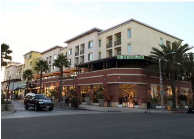
Example of a mixed-use building that provides an active street front and a stepback design to upper floors with residential uses.
