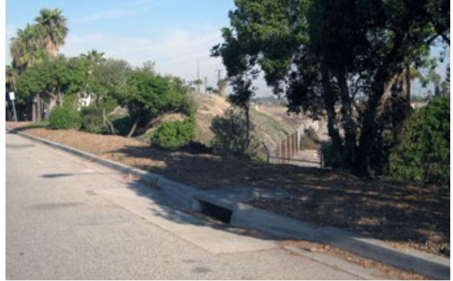
Infrastructure to support stormwater management is visible throughout the SEASP area.
