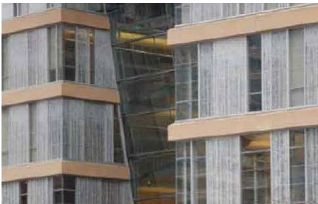
Angled glass is a dramatic architectural feature that reduces reflections of habitat and sky. Source: Minnesota Central Library, City of San Francisco Standards for Bird-Safe Buildings
