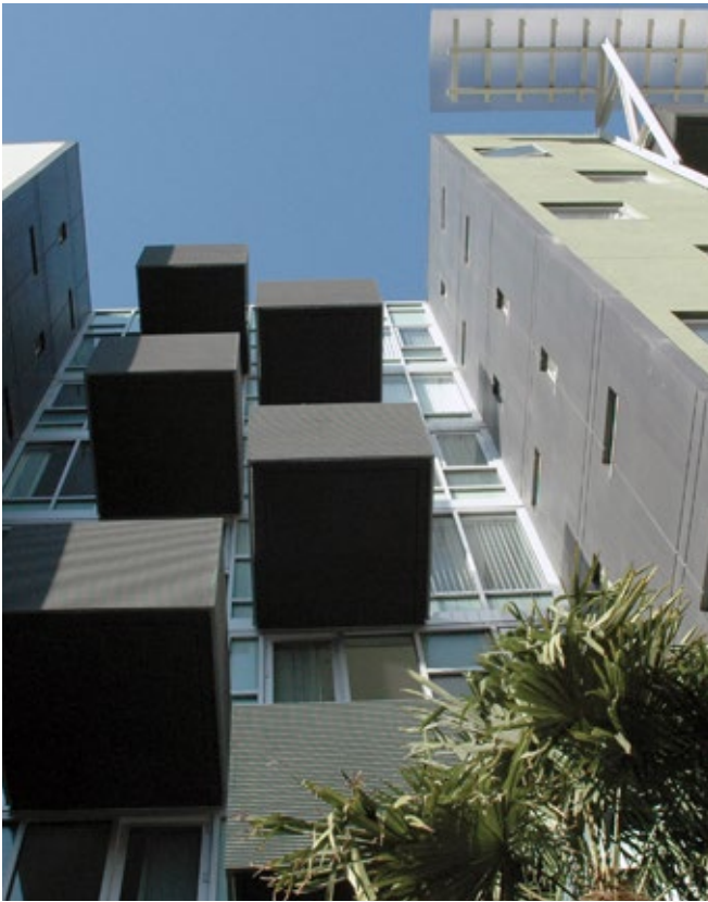
Balconies and overhangs can be used to block the view of glass from birds.
