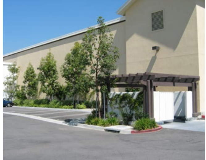
Pergola used to screen utility area.
