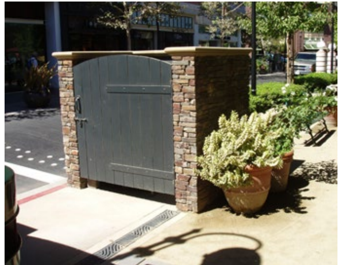
Brick and wood screen for utility area.
