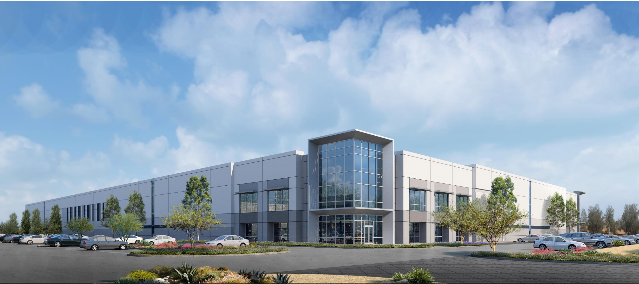
View of Building 2 looking northeast from Redondo Ave.
