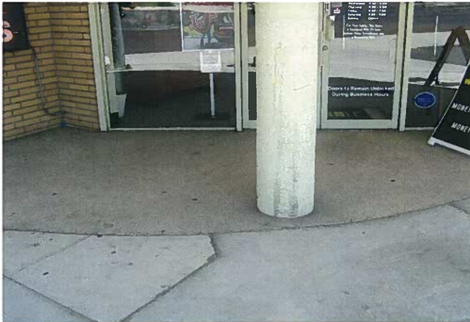
26 EXTERIOR-SIDEWALK & COLUMN AT ENTRY
