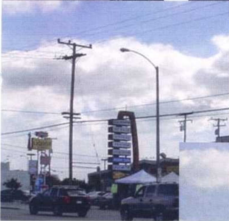
Dense aerial utilities on the south side of Willow Street west of the River on a busy commercial street.
