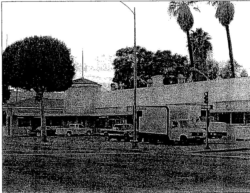
Primary (south and east) elevations, looking northwest.
