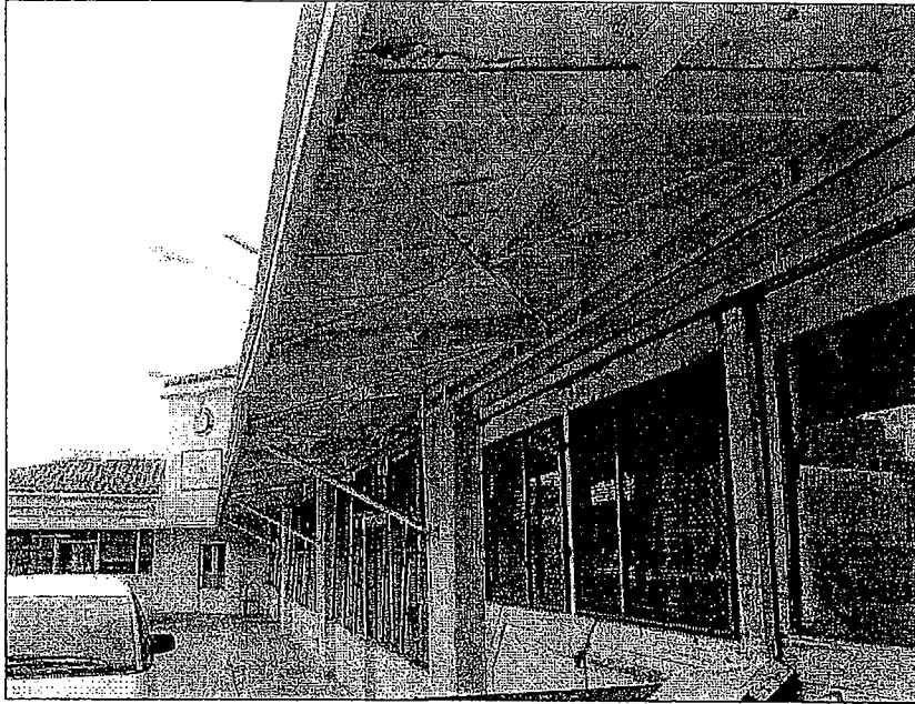
South elevation, north wing, looking west.
