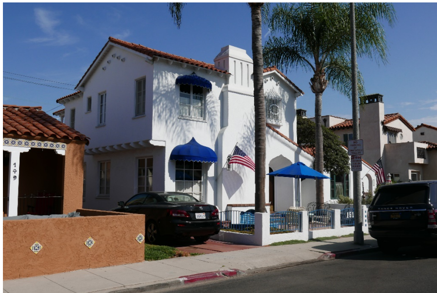
View of Primary (Eastern) Façade, 151 Saint Joseph Avenue
