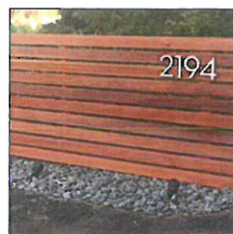
WD-1 WOOD SIDING CEDAR WITH CLEAR COAT
