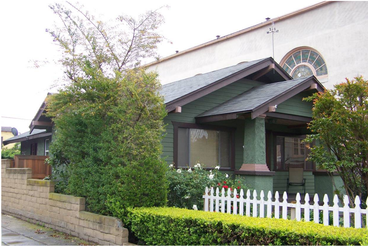
North and West Elevations Looking Southeast
