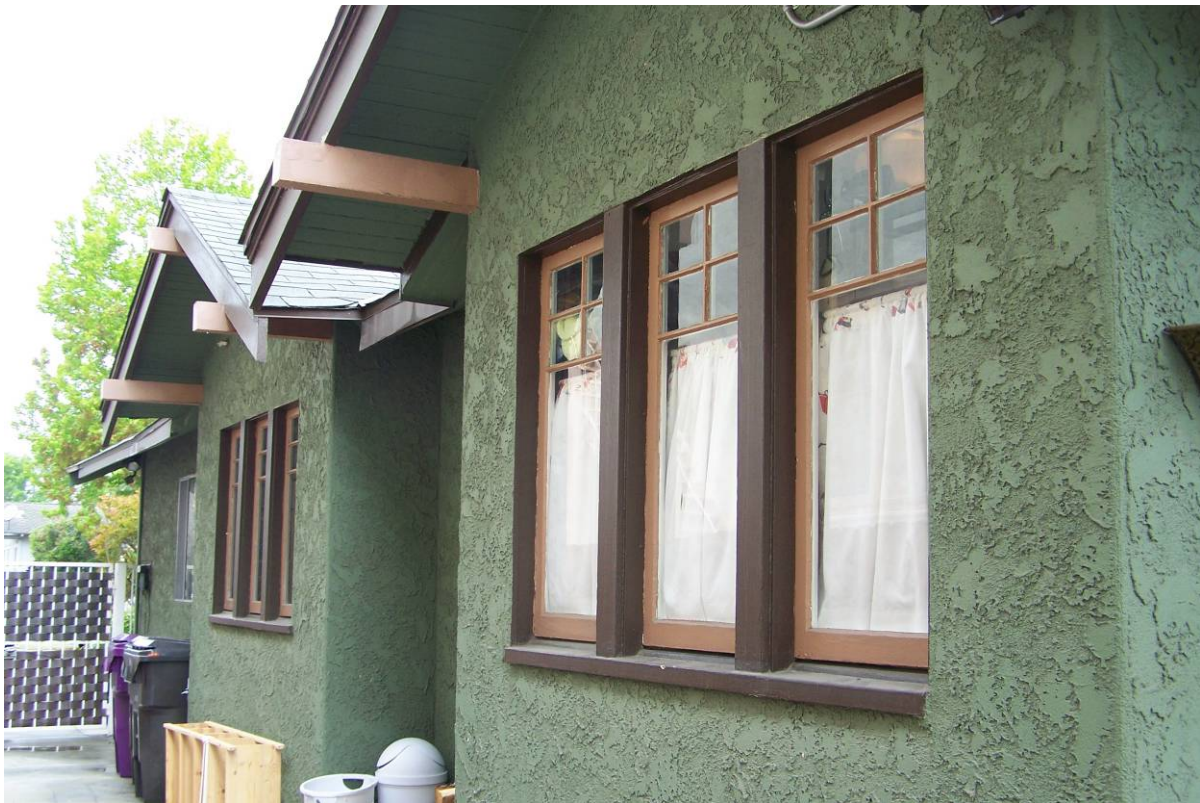
Detail of Wood Windows on South Elevation
