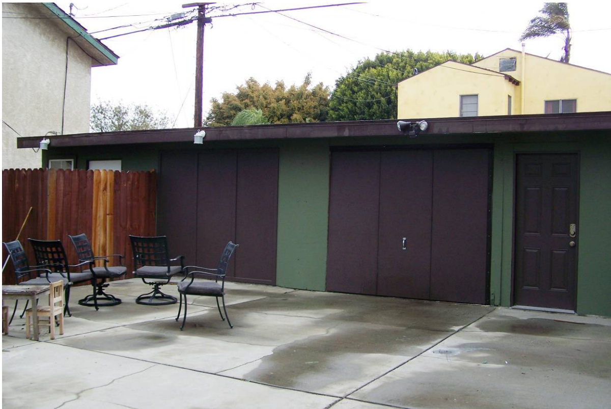
Auxiliary Building, West Elevation Looking East
