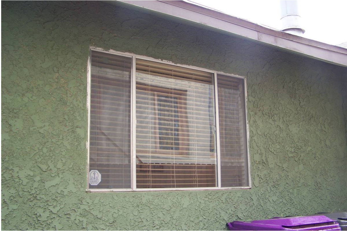
Detail of Aluminum Window on South Elevation
