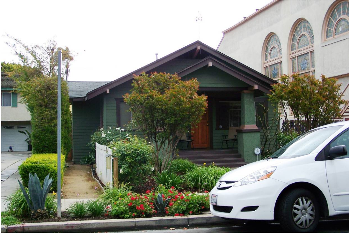
West Elevation Looking East
