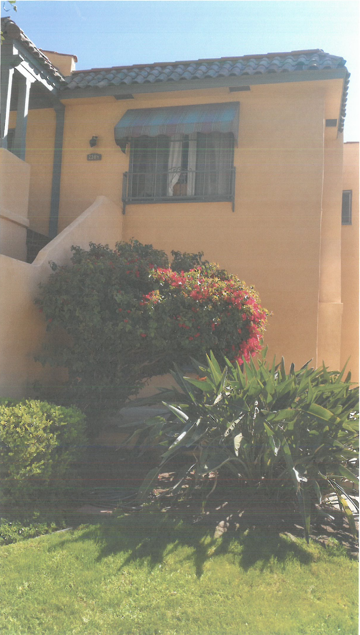
238 Coronado Ave. CB Overall view of front
